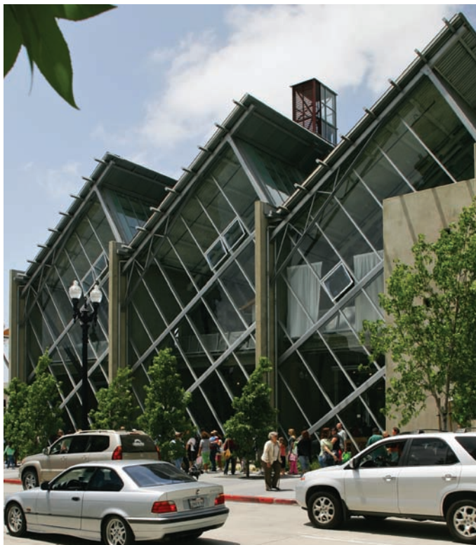
Photovoltaic panels on slanted roof segments are barely visible on The New Children's Museum. The central glass chimney seen on top serves as a cooling tower, exhausting hot air from gallery spaces.
